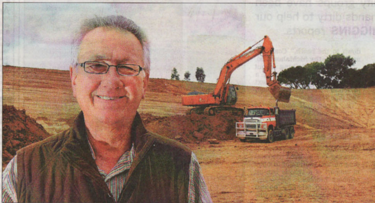
PROJECT: Willunga Basin Water Company chairman Norman Doole at the dam site. Picture: Helen Orr GUI26747
